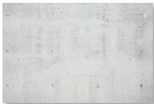
concrete & aerated concrete
